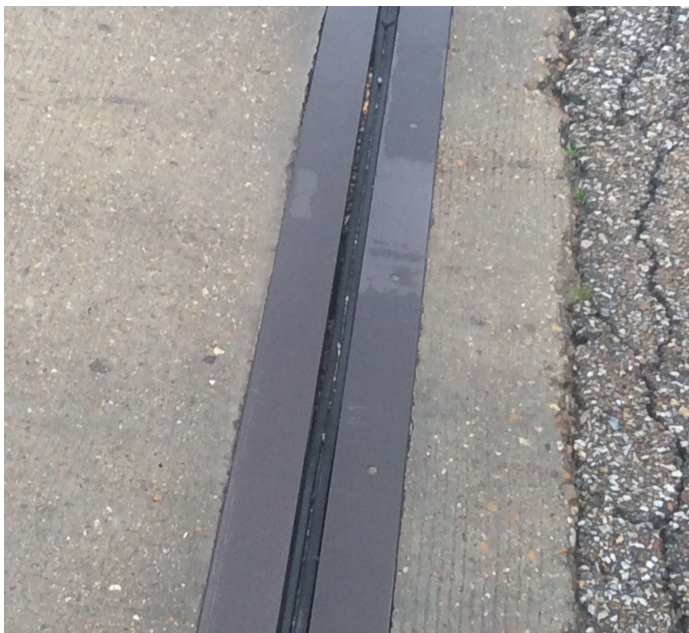
PHOTO 3 Description Joint seal leaking bent 1 north bound lane
