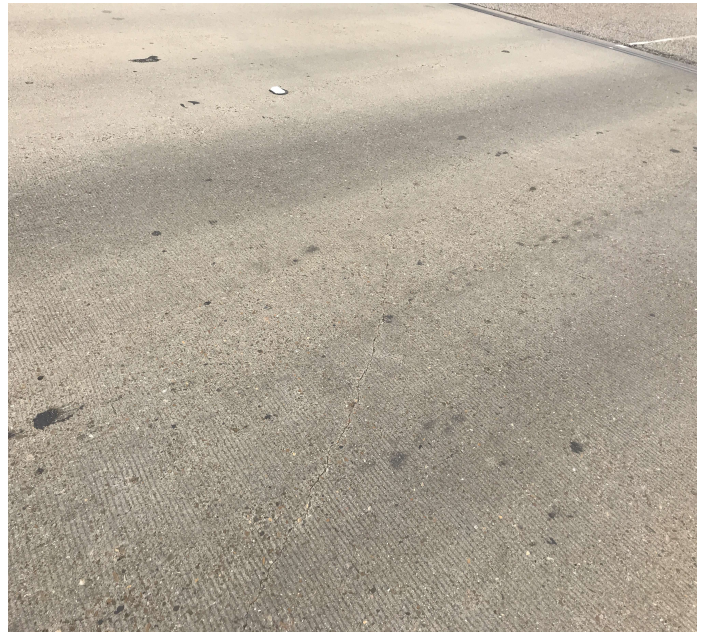
PHOTO 2 Description Span 1 northbound lane has large cracking in deck.
