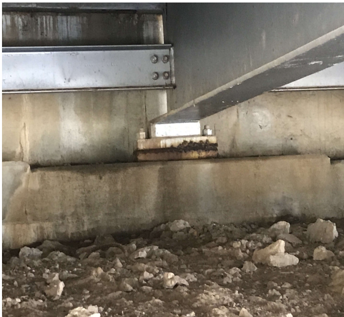
PHOTO 1 Description Bent 4 bearing 9 has flaking rust due to leaking joint seals.
