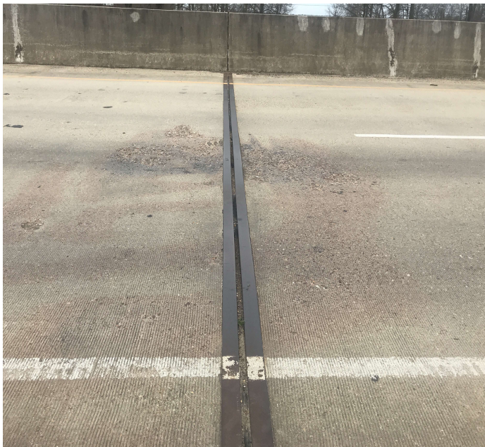
PHOTO 1 Description Bent 2 north bound lane joint seal has debris impacting loss of adhesion and are leaking.( Common on bent 3 also on North bound sides).
