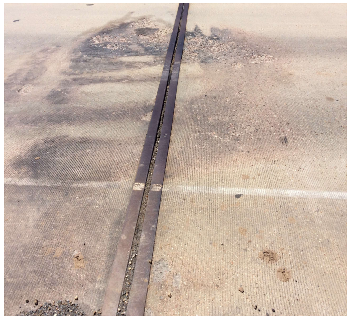
PHOTO 2 Description Deck - Bent 2 left side (northbound lanes): Fire damage
