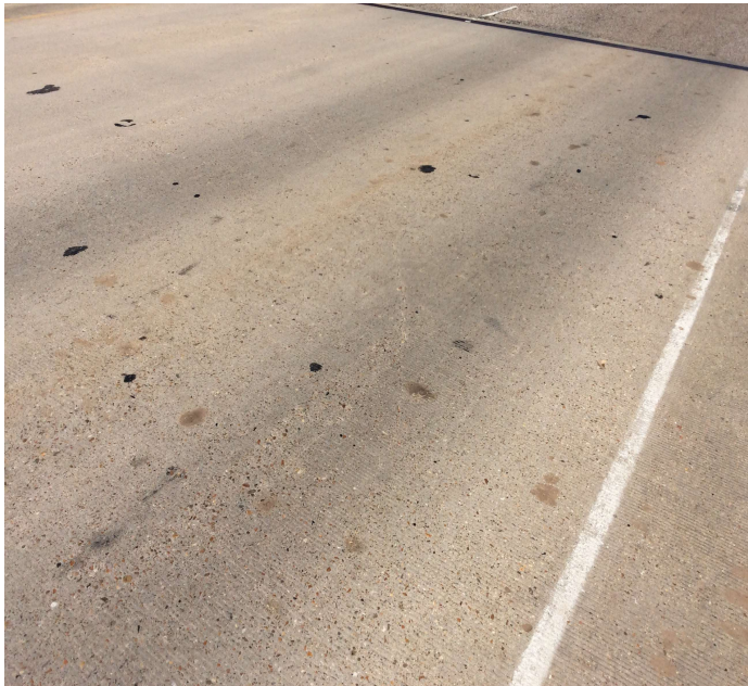
PHOTO 1 Description Span 1 left Typical cracking
