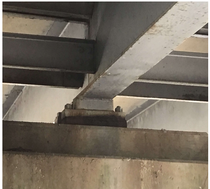
PHOTO 2 Description Bent 2 bearing 9 has heavy corrosion.
