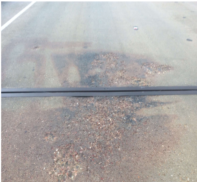
PHOTO 4 Description Fire damage northbound bents 1&2
