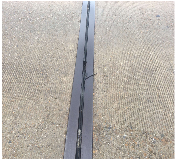
PHOTO 2 Description Bent 2 as approach south bound expansion seal torn and leaking
